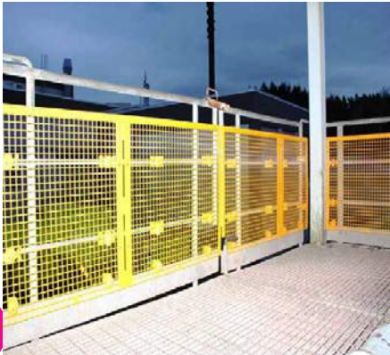
BLH Stop Drop™ Barricading installed on Platforms
