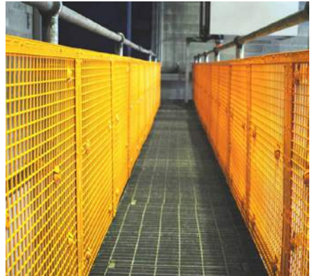
BLH Stop Drop™ Barricading installed on Walkways
